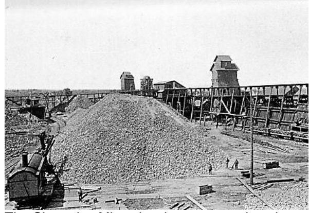
The Champion Mine showing a power shovel used for loading rail cars from the stockpile. The ore cars were destined for the ore docks in Marquette.
