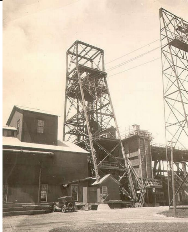
The Ludington Shaft headframe at the Chapin Mine.
