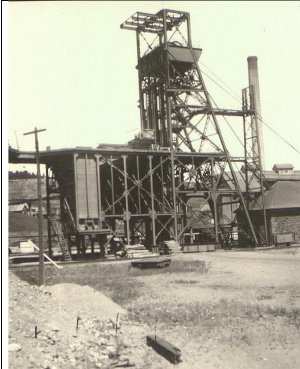
The Hamilton Shaft headframe at the Chapin Mine.
