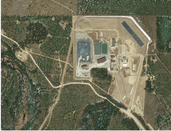
Aerial view of the Eagle Mine surface facilities (Google Earth, 2014 image)
