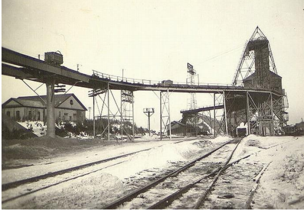
The Negaunee Mine with trestles for stockpiling ores by different chemical analyses.
