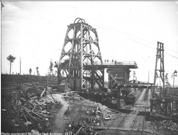
The Pewabic Mine headframe in Iron Mountain. Block caving was first used at this mine.
