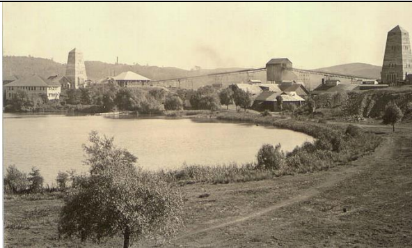
(Above) the two Cliffs Shaft Mine concrete, Egyptian Revival obelisk headframes (ca1919).
