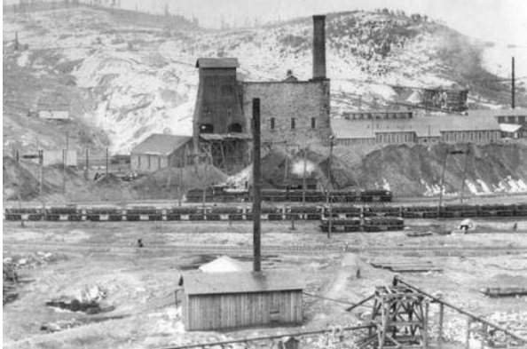
(Above) The Chapin Mine in Iron Mountain, Michigan used a huge pumping engine (right) to dewater the mine. It was housed in a 4-story stone, Cornish-style engine house. The engine has been preserved; however, the original engine house was demolished.
