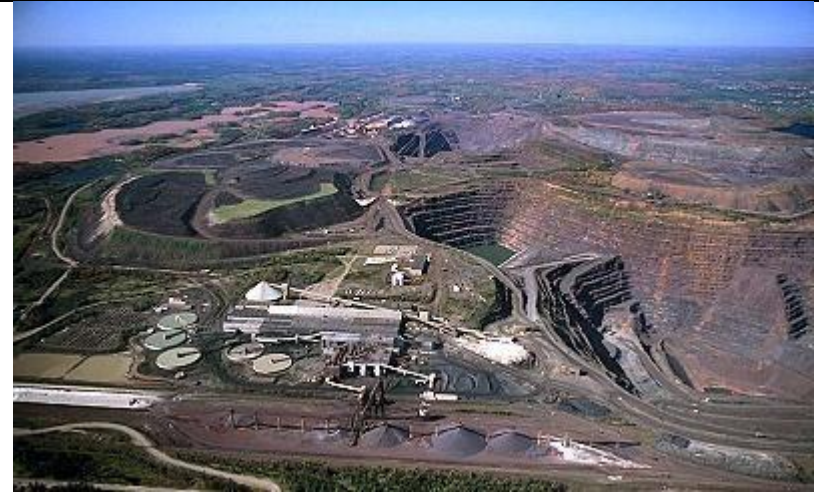
The Tilden Mine with concentrator and pellet plant. The Empire Mine, now closed, is in the far distance. (Courtesy Cliffs Natural Resources)
