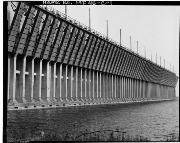
Concrete No. 6 Ore Dock, Marquette, Michigan, 1932. (HAER, Library of Congress)
